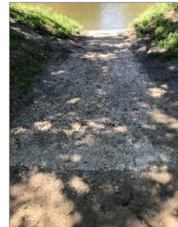
GRAVEL BOAT RAMP SURFACE
