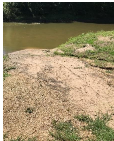
EXISTING ACCESS RAMP
